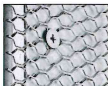
Wire lath to steel or wood studs.
